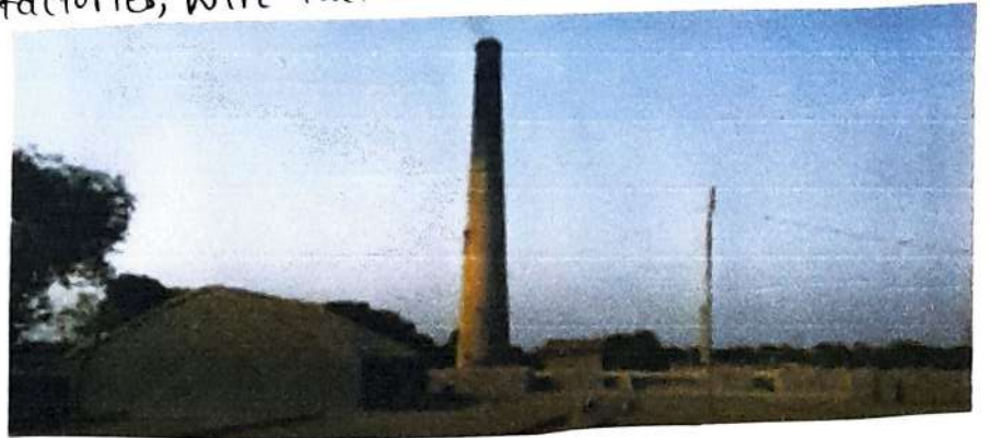
Brick manufacturing factory.
